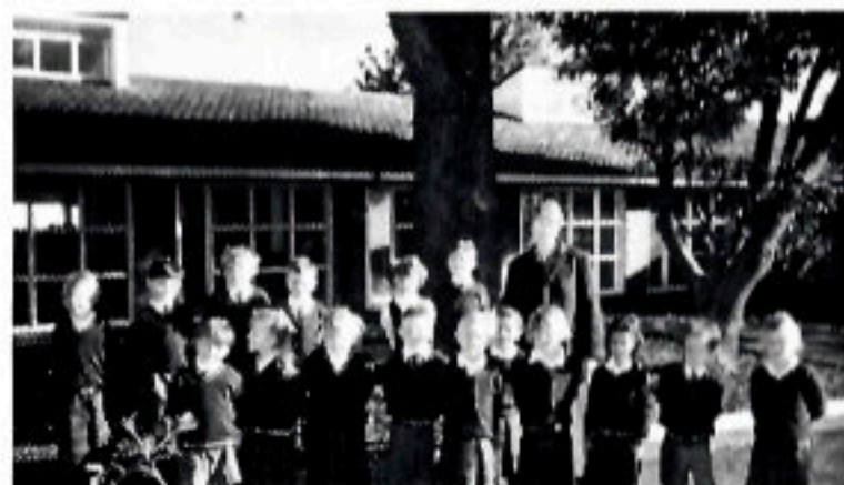
Mrs Brickland and Class One outside new classrooms.
